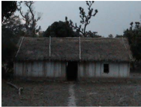
Figure 1.1.: Vulture Centre before renovation outside
