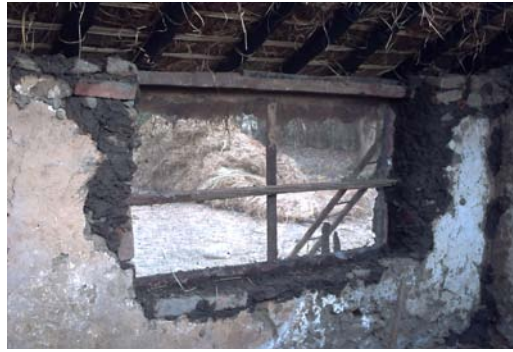
Figure 1.10.: Putting in of the window
