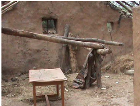
Figure 1.2.: Vulture Centre before renovation inside
